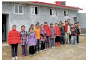
Newly built biogas toilet in local school. 新增務村小學沼氣生態廁所。
